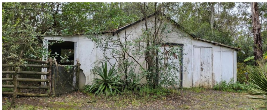
Image A2.16. Garage built in 1946 showing broken fibro sheeting next to the door opening at left ('3' in site plan in Image 1.1) (BHHH, 2024).
